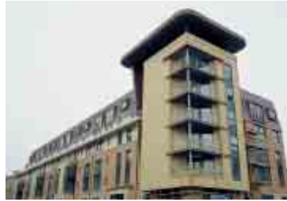
Two Berkely Street, Glasgow.
