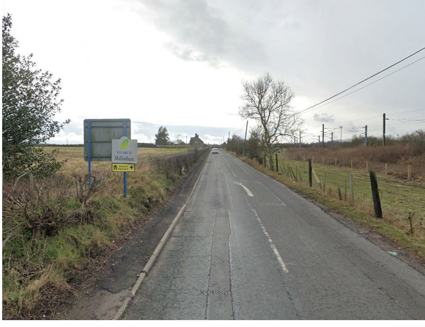
(02) Road closure Entrance facing east Old Craighall Road
