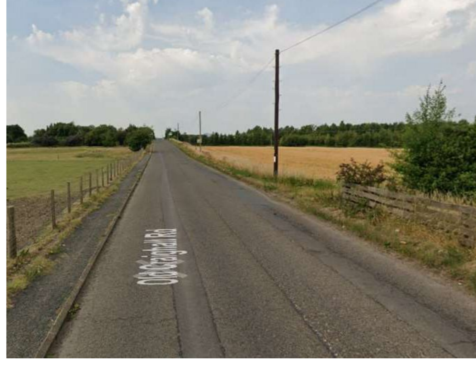
(04) View west along towards railway crossing, single sided pavement
