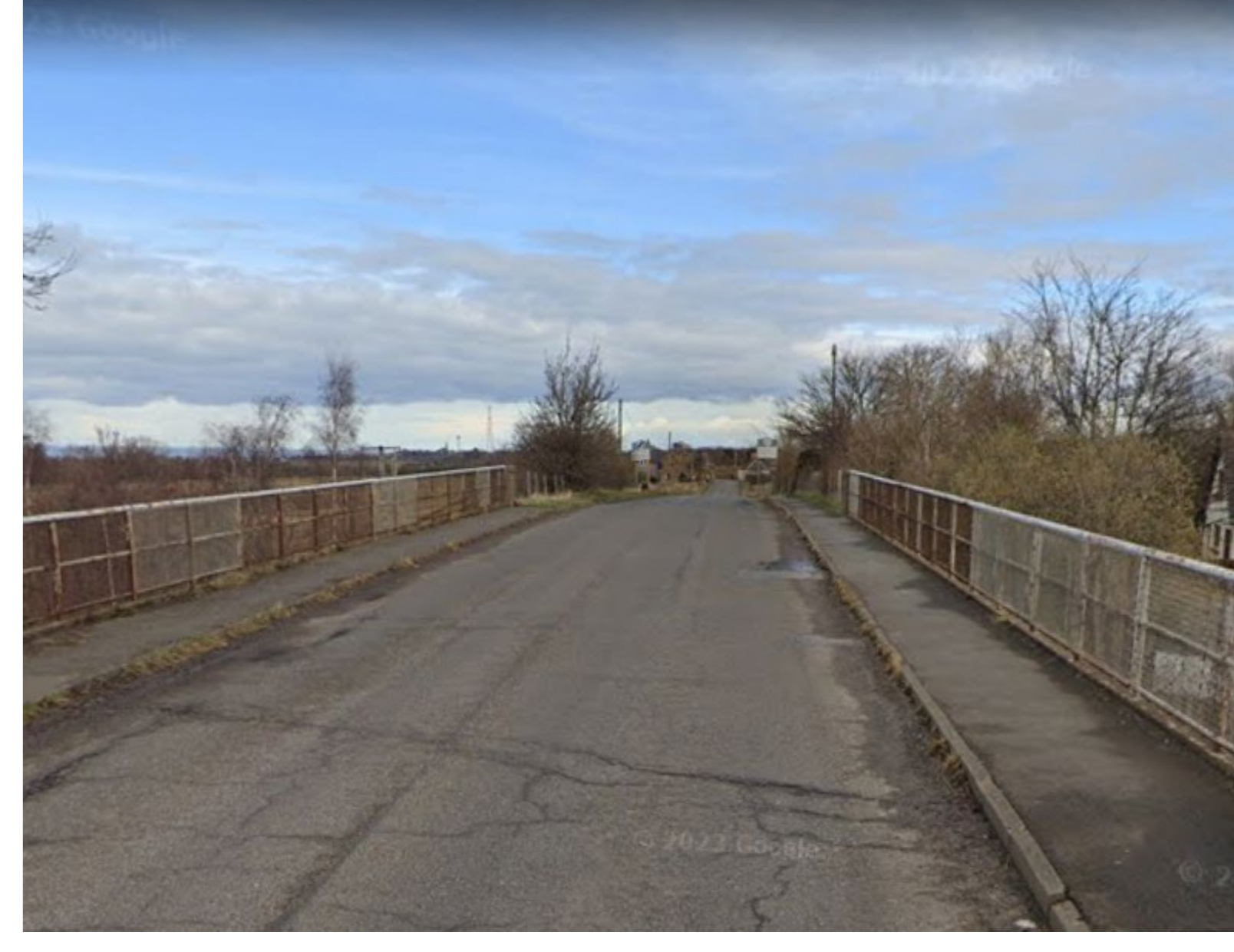
(05) View looking East from rail bridge along Old Craighall Road.
